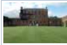
Mansion House Hall Place
